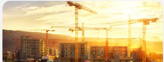
CONSTRUCTION, REMEDIATION, DEMOLITION
